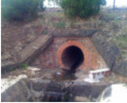
Railway culvert, Station Street
