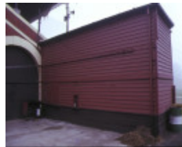
queen elizabeth oval grandstand bendigo entrance
