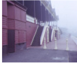
queen elizabeth oval grandstand bendigo front stairs
