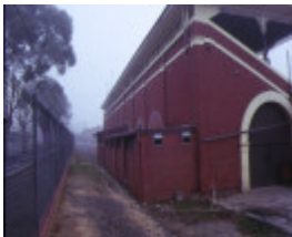
queen elizabeth oval grandstand bendigo rear view
