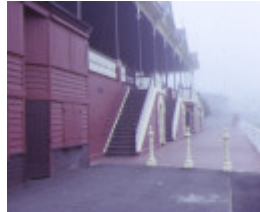
queen elizabeth oval grandstand bendigo front stairs
