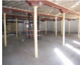
61-9 A'Beckett St ground floor MZ 24 05 2007
