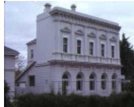
1 commercial banking co of sydney ltd bendigo front view
