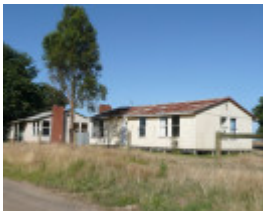
FORMER BALLARAT RAAF BASE SOHE 2008
