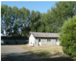
FORMER BALLARAT RAAF BASE SOHE 2008
