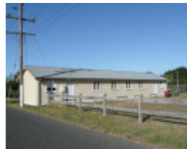
FORMER BALLARAT RAAF BASE SOHE 2008
