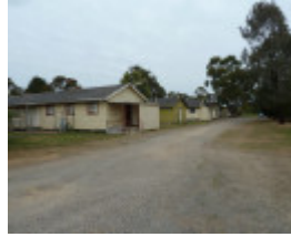
H2113 FORMER BALLARAT RAAF BASE LHA 2015 1.JPG
