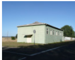
FORMER BALLARAT RAAF BASE SOHE 2008
