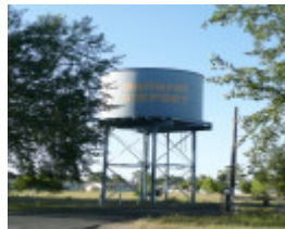
FORMER BALLARAT RAAF BASE SOHE 2008
