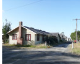
FORMER BALLARAT RAAF BASE SOHE 2008
