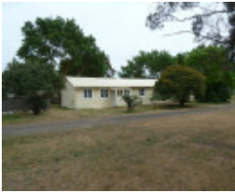
H2113 FORMER BALLARAT RAAF BASE LHA 2015 5.JPG
