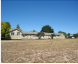
14247 Former Ballarat RAAF Base Admin building
