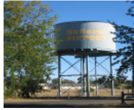
14247 Former Ballarat RAAF Base water tower
