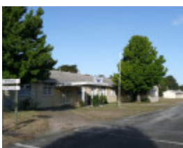
FORMER BALLARAT RAAF BASE SOHE 2008
