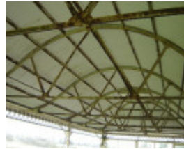
14252 Hamilton racecourse 4Sept06 grandstand roof
