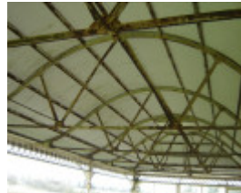
14252 Hamilton racecourse 4Sept06 grandstand roof
