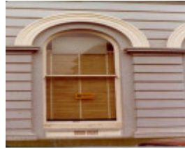
former bank of nsw view street bendigo window detail
