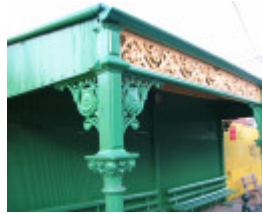
TRAM VERANDAH SHELTER SOHE 2008
