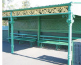
TRAM VERANDAH SHELTER SOHE 2008
