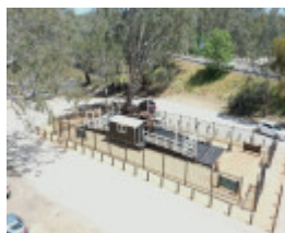
Barmah Punt LHGP Works Completed 2019
