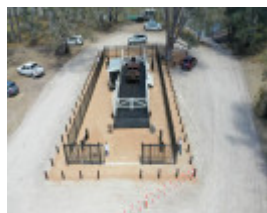
Barmah Punt LHGP Works Completed 2019 2
