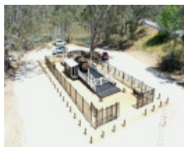
Barmah Punt LHGP Works Completed 2019 3
