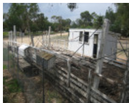
Barmah Punt_Barmah_Feb 2008_mz_Deck and Engine House 02
