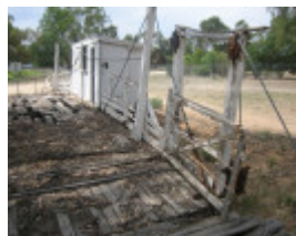
Barmah Punt_Barmah_Feb 2008_mz_Deck and Engine House
