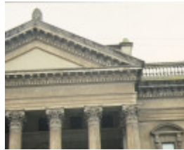
masonic hall bendigo detail pediment
