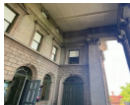
2023. Inside entrance portico, view of Corinthian column.
