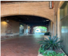
2023. Ground level right of way to ground floor of 1890 extension.
