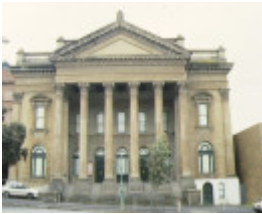
1 masonic hall bendigo front view
