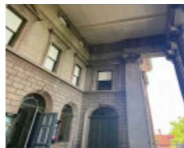
2023. Inside entrance portico, view of Corinthian column.
