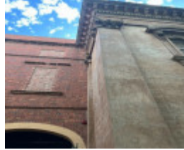
2023. Interface between original building and 1890 extension. 1890 extension was never rendered.
