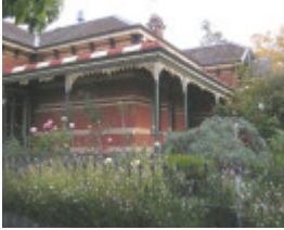
Review of C* Grade Buildings in the Former City of Hawthorn
