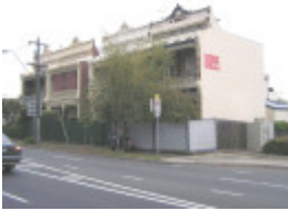
Review of C* Grade Buildings in the Former City of Hawthorn
