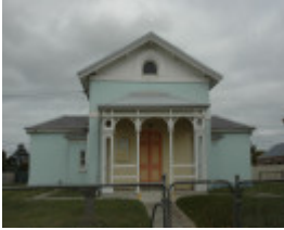
Former Ballan Court House, Moorabool Shire Heritage Study Stage 1, 2010
