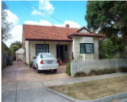
House at 6 Elliston St
