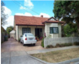
House at 6 Elliston St
