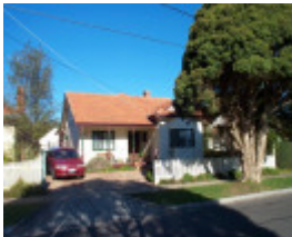
House at 6 Elliston St
