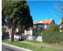
House at 6 Elliston St
