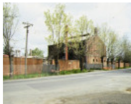
1 former bendigo gas works bendigo rear view oct1992
