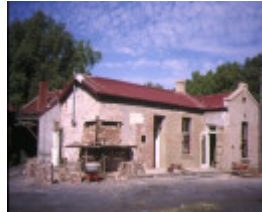
former bendigo gas works bendigo residence office
