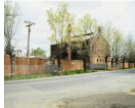
1 former bendigo gas works bendigo rear view oct1992
