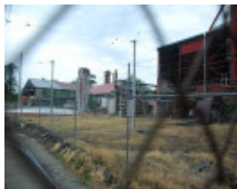
FORMER BENDIGO GAS WORKS SOHE 2008
