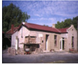
former bendigo gas works bendigo residence office
