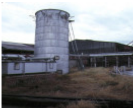
former bendigo gas works bendigo silo mar1989
