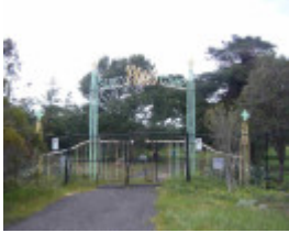
'The Pines' Scout Camp, Hobsons Bay Heritage Study 2006 - The cover image shows the entrance gates and archway erected in 1964.
