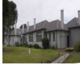
Altona Primary School No. 3923 Complex and trees, Hobsons Bay Heritage Study 2006 - image shows the 1922 school (left) and 1926 additions.
