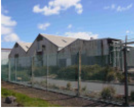
Shell Oil Complex, Hobsons Bay Heritage Study 2006
