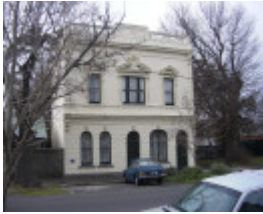
George Hotel (former), Hobsons Bay Heritage Study 2006
