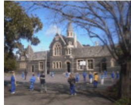
Williamstown Primary School No. 1183, Hobsons Bay Heritage Study 2006 - image shows another view of the school, framed by trees including a Moreton Bay Fig (left) and a Dutch Elm (right) along the Cecil Street frontage.
