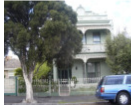
160 Cecil Street, Hobsons Bay Heritage Study 2006
