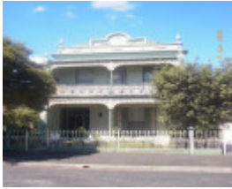
160 Cecil Street, Hobsons Bay Heritage Study 2006
