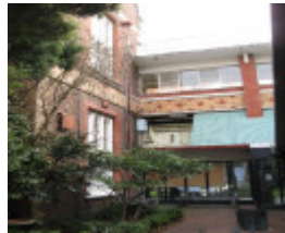
Alfred Hospital Aug 26 2011 KJ east side.jpg
