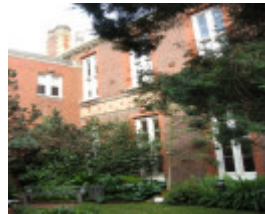
Alfred Hospital Aug 26 2011 KJ east side.jpg
