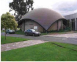
Altona Civic Offices Council Chambers (former), Hobsons Bay Heritage Study 2006
