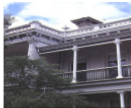
rochester terrace st vincent place albert park balcony
