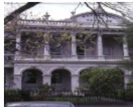
rochester terrace st vincent place albert park central balcony detail
