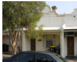
10-16 Davies Street, Hobsons Bay 2006/2007 precinct images No 14
