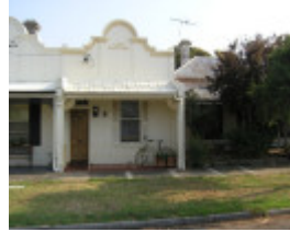
10-16 Davies Street, Hobsons Bay 2006/2007 precinct images No 10
