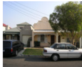
10-16 Davies Street, Hobsons Bay 2006/2007 precinct images No 16
