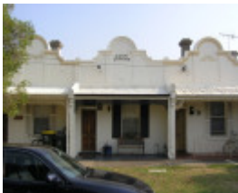
10-16 Davies Street, Hobsons Bay 2006/2007 precinct images No 12
