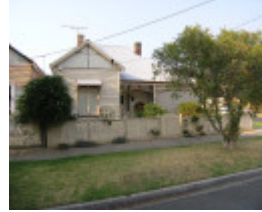
10-16 Davies Street, Hobsons Bay 2006/2007 precinct images No 11
