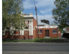
Excelsior Lodge of Industry Masonic Temple, Hobsons Bay Heritage Study 2006
