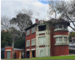
526 Punt Road South Yarra
