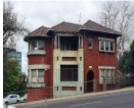
526 Punt Road South Yarra
