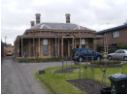
House at 92 Esplanade WILLIAMSTOWN, Hobsons Bay Heritage Study 2006
