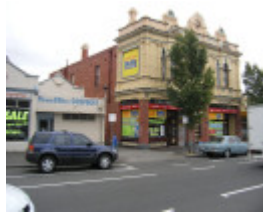
Punshon's Federal Stores (Former), Hobsons Bay Heritage Study 2006
