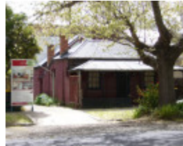
House at 46 Hanmer Street WILLIAMSTOWN, Hobsons Bay Heritage Study 2006
