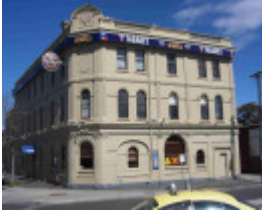
Newport Hotel (former), Hobsons Bay Heritage Study 2006
