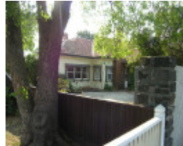
House at 278 and 280 Melbourne Road NEWPORT, Hobsons Bay Heritage Study 2006 - No 278
