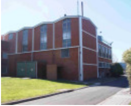
MMBW Brooklyn Pumping Station, Hobsons Bay Heritage Study 2006
