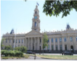
SOUTH MELBOURNE TOWN HALL SOHE 2008
