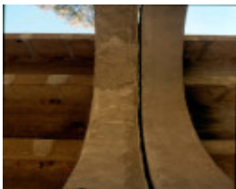
H01986 janevale bridge underside expansion joint jan02
