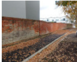
Wall along Stawell Street
