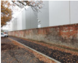
Wall along Stawell Street
