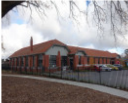
Former Toddlers' Block (2025)
