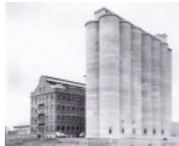
c 1940 depicting the south-west fa ade of the complex including the 1926-7 storehouse and mill building and the 1939 reinforced concrete silos
