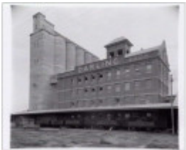
c 1940 depicting the east fa ade of the complex including the 1926-7 mill building rail siding loading platform canopy and rail cars and the 1939 concrete silos
