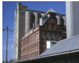
john darling & son flour mill albion silos
