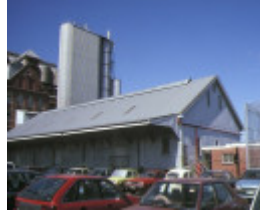
john darling & son flour mill albion delivery building
