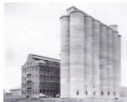
c 1940 depicting the south-west fa ade of the complex including the 1926-7 storehouse and mill building and the 1939 reinforced concrete silos
