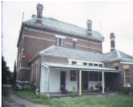
kiora south road brighton rear view nov1985
