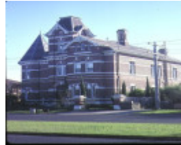
1 kiora south road brighton side view jun1981
