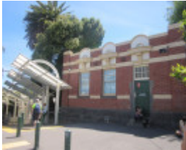
Essendon Railway Complex (Russell Street Entrance).JPG
