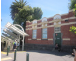
Essendon Railway Complex (Russell Street Entrance).JPG
