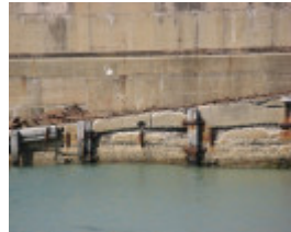
Warrnambool breakwater_ mass concrete_KJ_May 09
