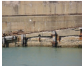
Warrnambool breakwater_ mass concrete_KJ_May 09
