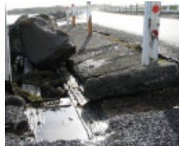
Warrnambool viaduct now_2009
