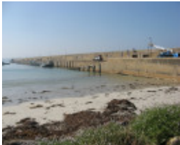
Warrnambool Concrete breakwater_KJ_May 09
