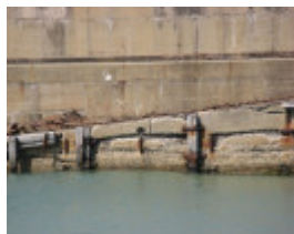
Warrnambool breakwater_ mass concrete_KJ_May 09
