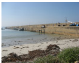
Warrnambool Concrete breakwater_KJ_May 09
