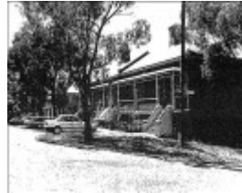
Fernville Terrace, 35-41 Mackenzie Street, 1885-; demonstrating the influence of the steep terrain on house design in this part of Bendigo where sub-basements become full height on the downhill side of a site.
