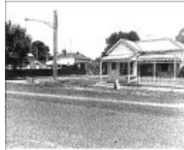
Precinct 6.04 - corner of Milroy and Stevenson, precinct 6.4: corner store and adjacent timber houses of the late 19th early 20th centuries.
