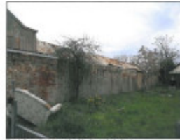
Photo 1: Rear wall of former brewery building.
