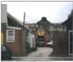
Photo 5: Section of original brewery building.
