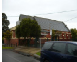
Parish Hall & Club Room (Former)
