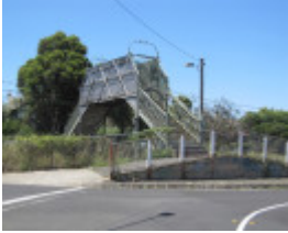
Eglinton Street Pedestrian Bridge.JPG
