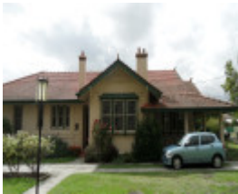
St Mary's Presbytery, west side
