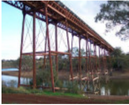
Melton Viaduct - Over the Melton Weir MELTON SOUTH, MELTON SHIRE
