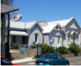
H543 orderly room residence kepler st1
