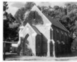
St Stephen's Anglican Church John Collins 1982 SLV
