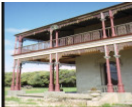
fairfield murray hwy browns plains verandah of homestead sep1990
